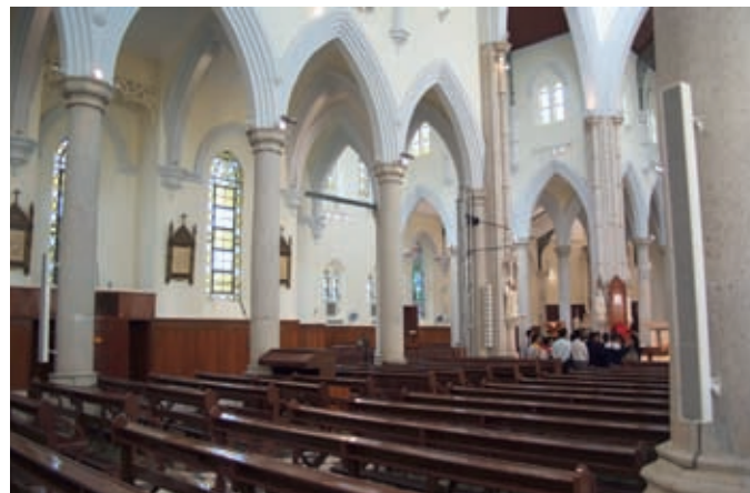
Final installation of the loudspeaker columns
